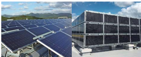
Solar power generation (located not only on the rooftop, but also installed vertically as blind walls)
