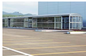
Arcade and snow-melting system installed in the parking lot
