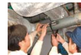
Performing energy measurements at a manufacturing site (October 2009)
