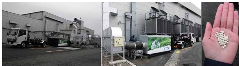
Heat storage using thermal storage materials at the exhaust heat site
