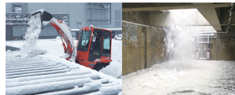
Snow use pit (left: Input port; right: pit interior)
