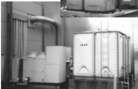
Thermal storage air conditioning system at the D3 wing of the Narita Plant
